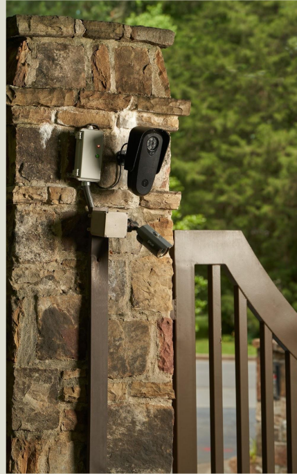
Electric & Existing Structure / Pole
